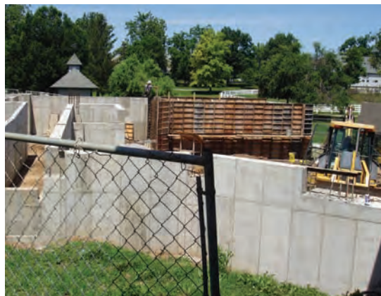
Construction as of July 17, 2009.
