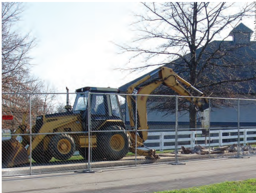
Showplace for Saddlebreds construction begins.
